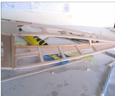
The photo of P6 in place
