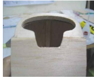
Align F13 with F0 (do not glue the front of F13 to F0)
